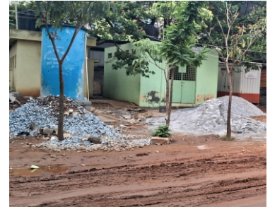
Identified place for construction of one block
