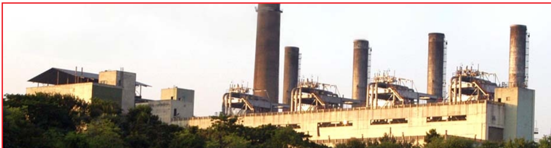
Bandel Thermal Power Plant, West Bengal
