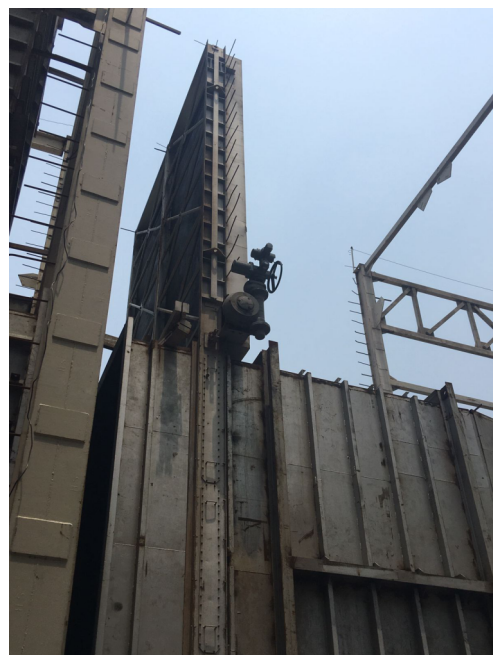
Commissioning of Auma SIL actuator at site
