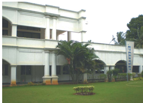
Auma India Manufacturing Unit at Peenya
