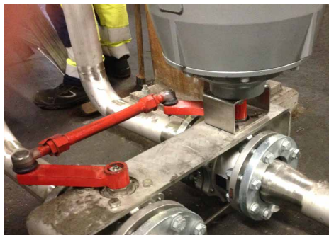
Each of the two AUMA fail safe actuators drives a pair of cooling water valves in tandem.
