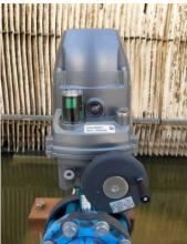
196 compact and smart **PROFOX** actuators have replaced old, error-prone pneumatic actuators in the district cooling plant in Palm Jumeirah. AUMA took care of the entire retrofit project management.
