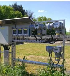
AUMA SAR 07.6 actuators are installed underground at Łyna wastewater treatment plant. AUMA's modular design allows their AC 01.2 actuator controls to be mounted accessibly at ground level.
