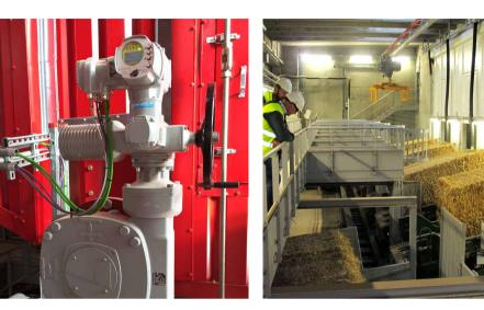
An AUMA SA actuator with AC 01.2 actuator controls in SIL version meets stringent SIL 2 requirements at Lisbjerg power plant.
