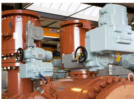
Fireproof shields for the SAEx actuators and ACExC 01.2 actuator controls ensure that the valves can operate reliably even in the event of a fire.
