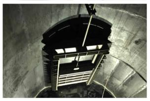
AUMA SA-UW actuators for continuous underwater use secure operation of underground emergency roller gates even when flooded.
