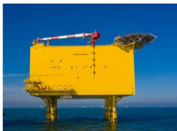
AUMA electric actuators are increasingly being deployed on offshore converter platforms providing high voltage direct current transmission (HVDC) for wind farms. Approximately 150 AUMA SQ part-turn actuators with intelligent AC actuator controls are, for example, installed on the BorWin gamma converter platform in the North Sea. AUMA will also supply actuators for the DolWin kappa platform. Both offshore platforms are owned by TenneT, one of the leading transmission system operators in Europe.
