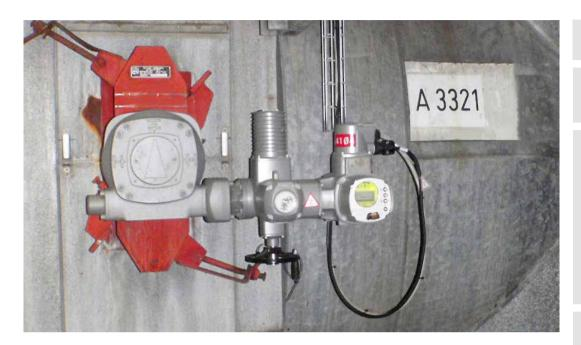
AUMA actuators that are TÜV-certified for use in safety related systems up to SIL 3 have proved a perfect fit as part of a safety system for flue gas scrubbers on an incineration plant installed at BASF in Ludwigshafen, Germany. At its headquarters in Ludwigshafen, Germany, BASF operates an incineration plant for the disposal of solid, pasty and liquid wastes created at BASF production sites. Flue gas from the incinerator is cleaned in a multi-step process that includes wet scrubbing.
